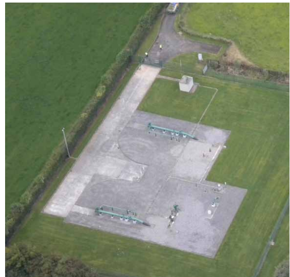
Figure 10.2 Aerial View of an AGI Site
